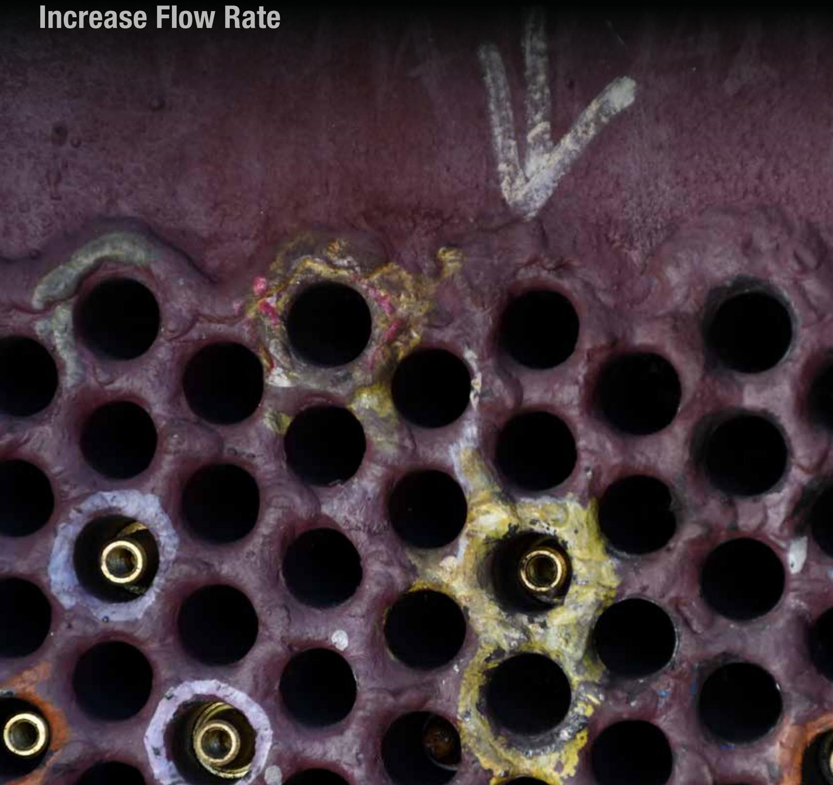
*This article relates a novel case-study use of tube plugs by the Dutch company Wilton Heat Transfer Services (formerly Bronswerk Heat Transfer Services) to solve a problem that an end-user client – a gas production and distribution company – were having with a heat exchanger in one of their process trains.*
