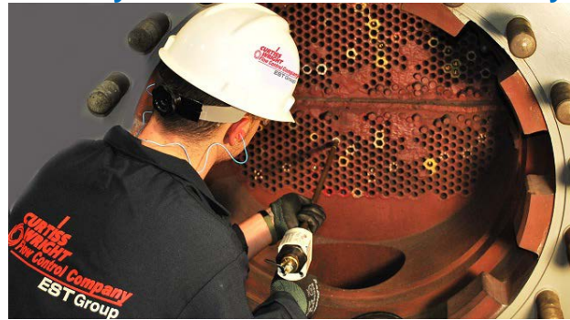
(Fig 2 Non Urea specific installation of Pop-A-Plug)
