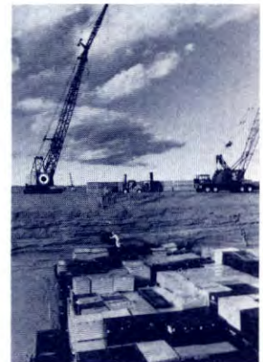
Figure 49. Low Level Waste Disposal Site. Waste containers are stacked in specially designed trenches. When full, the trenches are covered with soil and continuously monitored. (See close-up, Figure 50.)
