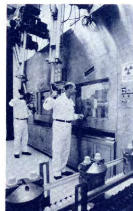
Figure 32. Shielding. Thick glass windows protect workers from radioactive materials in an industrial laboratory.
