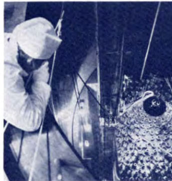
Figure 40. Lifting the Assembly. The crane used to move new assemblies into the reactor core also is used to move spent fuel from the reactor to the spent fuel pool.
