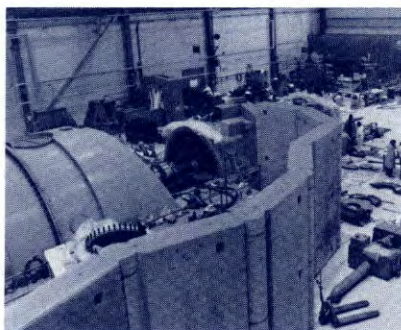
Figure 31. Shielding. This concrete wall around a BWR turbine reduces radiation exposure to surrounding areas.
